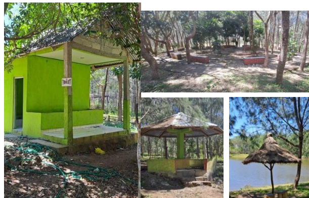
Figure 5. Facilities in Nifu Koko Reservoir
