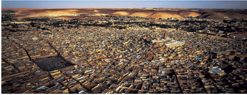
Figure 1: The architecture in the city of Ghardaïa
