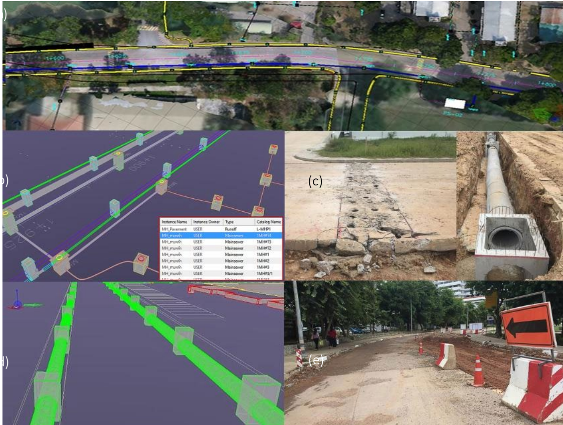
Figure 10: Integration of UIM in underground drainage pipe construction: (a) pipeline layout map showing connections and pipe positions; (b) intelligent model simulation of the drainage system with graphical and non-graphical data for planning and assessment; (c-e) stages of excavation and pipe installation.
