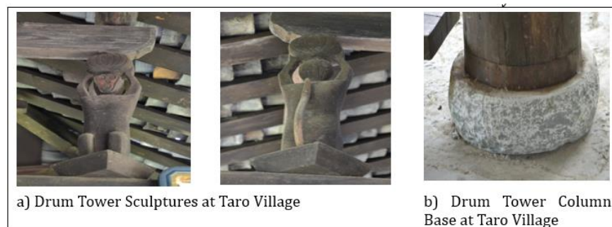
Figure Captions 9: Shows the Drum Tower Sculptures (a) and Drum Tower Column Base at Taro Dong Village
