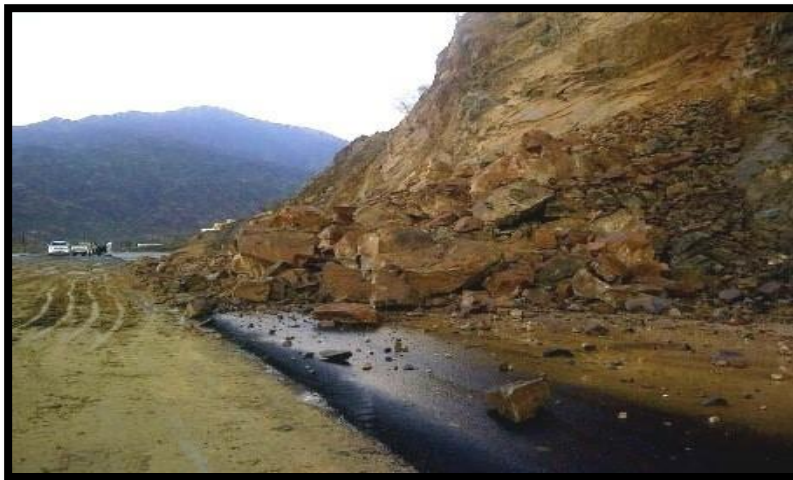
Figure 4: Rockfall in Kalar District
